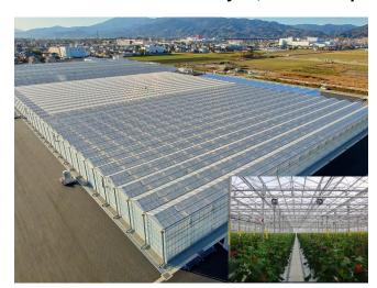
"Yume-Farm SAGA" completed last year Surface area: about 1 ha Dutch-light type, high-eave, steel-frame house (eave height: 5.0 m)
