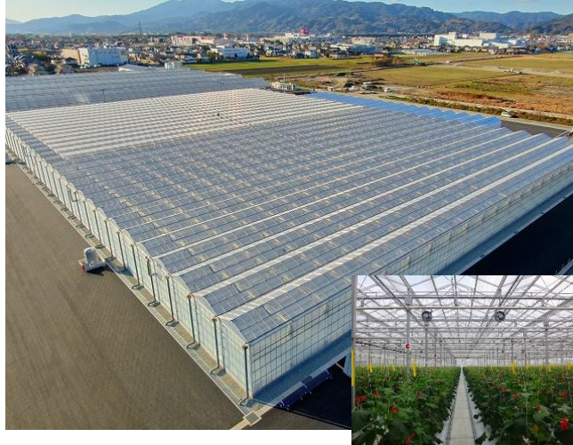
Surface area: about 1 ha Dutch-light type, high-eave, steel-frame house (eave height: 5.0 m)
