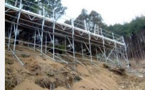
Disaster prevention work of Slope
