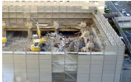
Demolition work Demolition works of structures accompanied by reconstruction, repair, etc.
