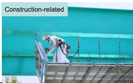
Construction-related Hanging type scaffolding (Spider Panel) Walking panel hung with chains, mainly used in bridge repair work
