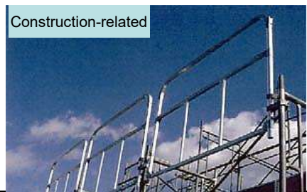
Construction-related Safety member Preceding handrails, baseboards, handrail members, etc.
