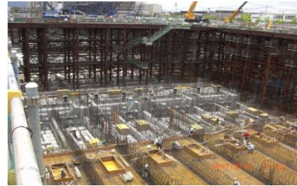
Plant Construction and maintenance of treatment plants, incineration facilities, plants, etc.
