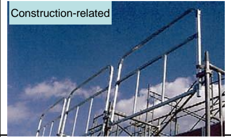
Safety member Preceding handrails, baseboards, handrail members, etc.
