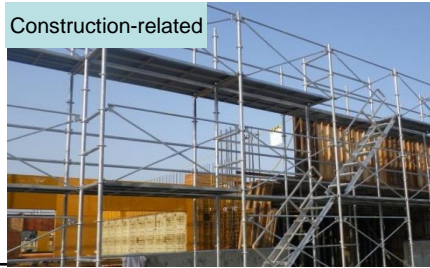
Next generation scaffolding (Iq system) New scaffolding with high safety performance, an alternative to the conventional building frames
