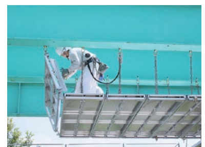
SPIDER PANEL, panel-type hanging scaffolding
