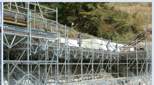
YT Lock System: Scaffolding system used for landslide prevention work
