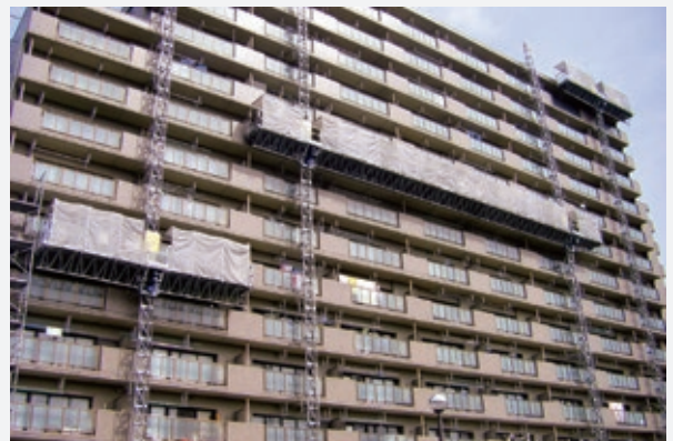
Renovation work on large-scale condominiums
