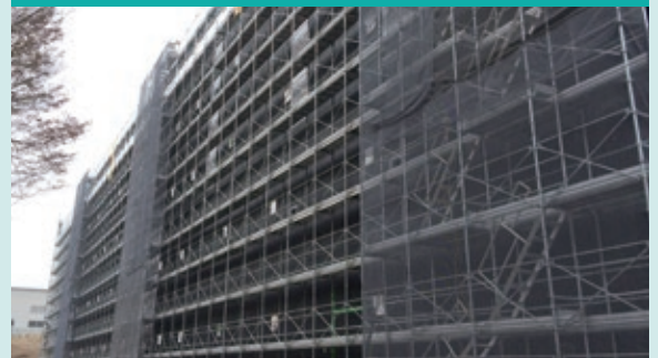
Scaffolding primarily set up around the exterior walls of construction
