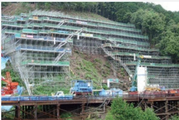
Scaffolding setup on slope
