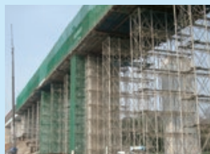
Falsework for construction of bridges in mountainous regions and viaducts
