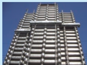
Mobile elevating scaffolding for use in the renovation of ultrahigh-rise buildings and towers
