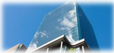
Grand Front Osaka Tower B 27th Floor
